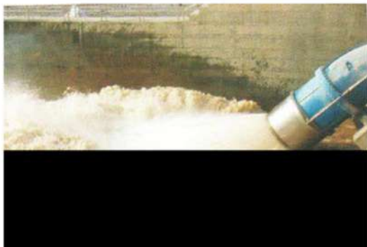
The oblique installation for energy dissipation
